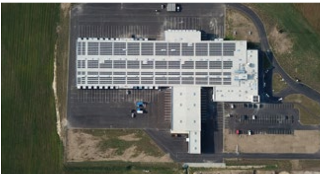
COMPACTFLAT, 500 KW, Estonia
