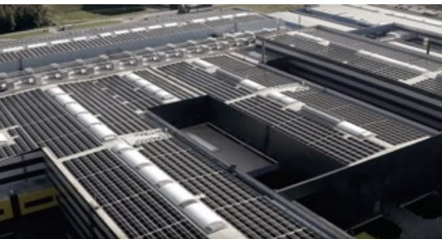
COMPACTFLAT, 6,9 MW, Austria
