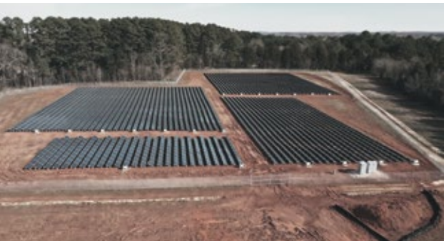
COMPACTGROUND, 1,3 MW, USA
