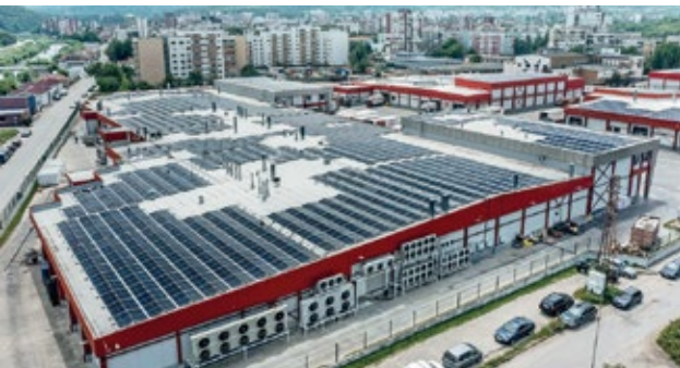
COMPACTFLAT, 1,779 kWp, Bulgaria
