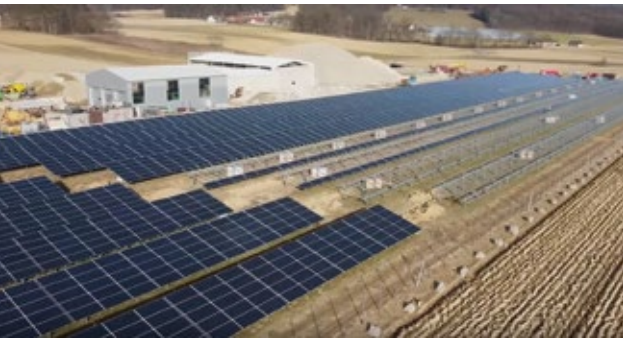
COMPACTGROUND, 3 MW, Austria
